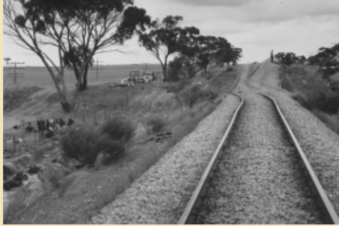
Meckering Earthquake Western Australia October 1968 21 injured and 35,000 people affected.
