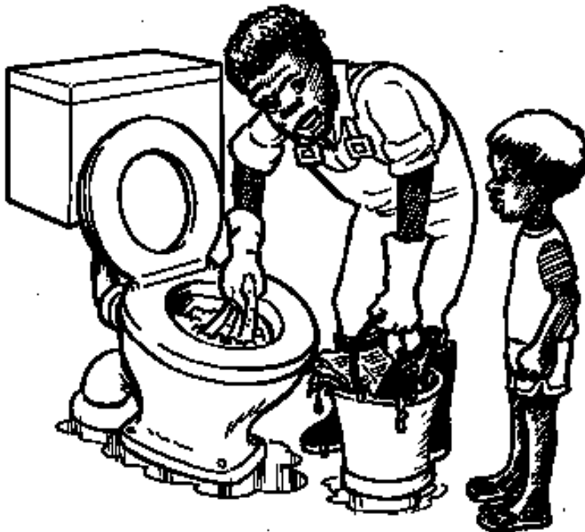
Fig 2.18: Toilets which are not working properly must be fixed.
