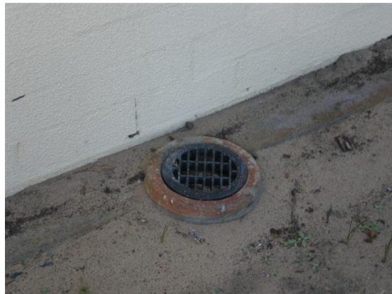
Overflow Relief Gully
